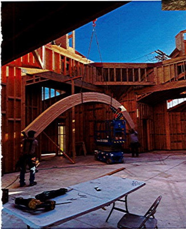
The construction of the new St. John the Baptizer Church has begun!
